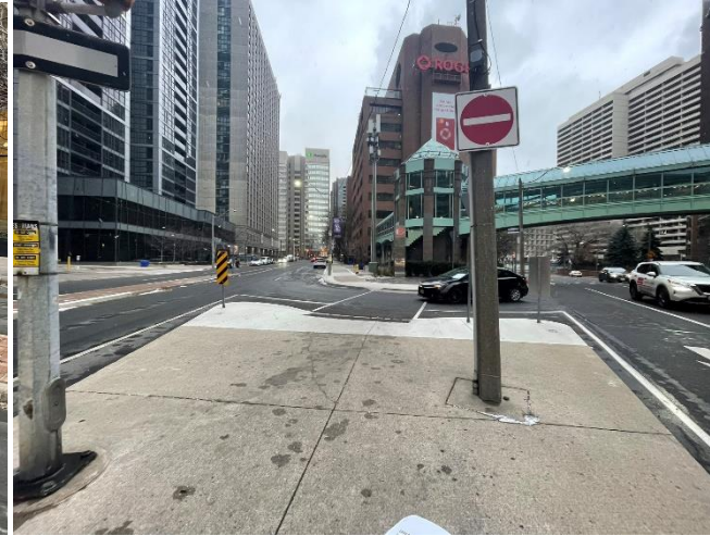
Channelized island at the Northeast corner of the intersection looking north towards Mount Pleasant and Ted Rogers Way.
