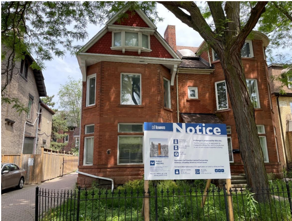
Exhibit C – Huntley and Earl Streets. Example of dwelling on Earl at closed intersection with Huntley Street, to be replaced with a 63-story condo tower.
